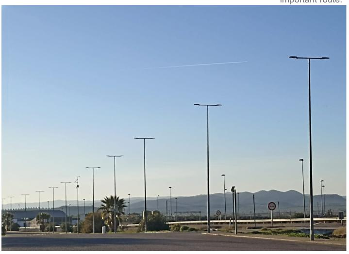
The town of Villafranca in Córdoba has undertaken a significant project to enhance the lighting of a heavily trafficked road. In order to ensure the safety of drivers and pedestrians, over 150 Milan S 60W luminaires have been installed along the road.
